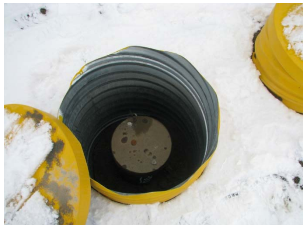
Figure 4.8. Typical Instrument Surface Completion Showing Outer 24-In.-Diameter Corrugated Metal Pipe Sleeving and Inner Steel Casing (Nest TA; photo taken in the winter 2008; snow can be seen on the ground)
