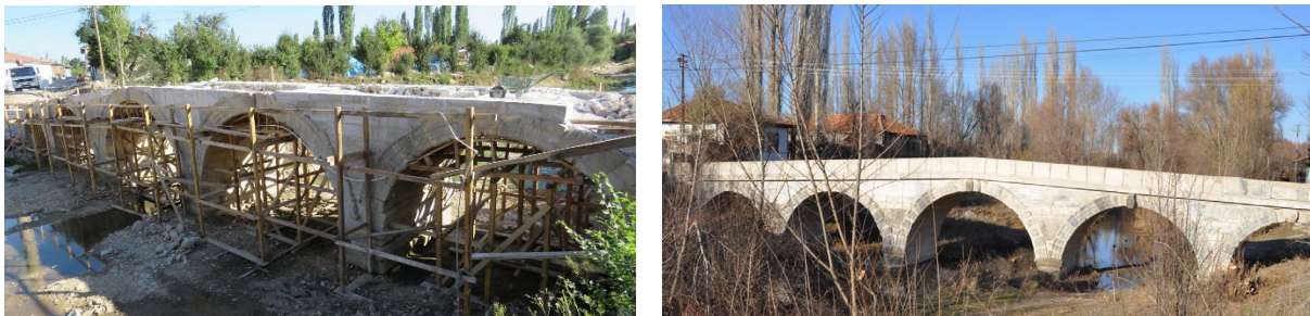
Figure 1. Pictures taken from during the restoration works
