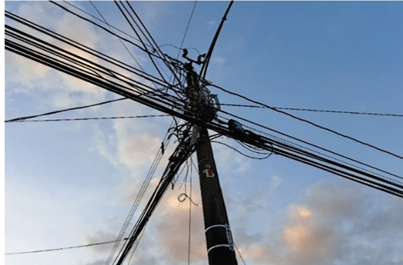
Figure 30: View of power and communications line systems in different directions, sharing the same space and infrastructure
