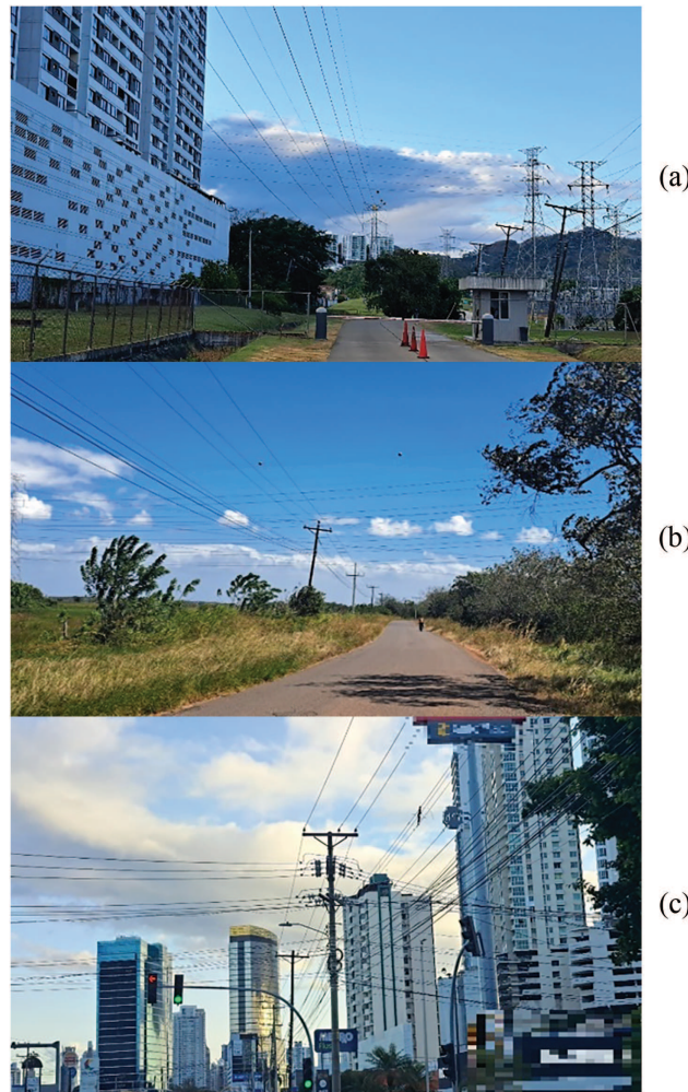
Figure 18: Situations of power line crossings are shown on: (a) two high voltage lines; (b) high voltage and medium voltage line; and (c) two medium voltage lines
