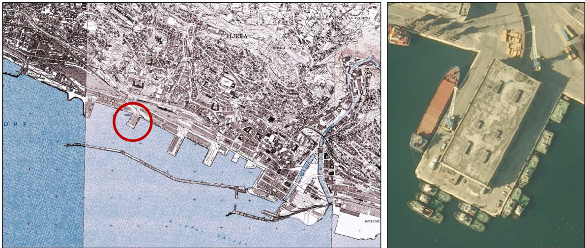
Figure 1: The Port of Rijeka with enlarged view of Warehouse no. 17 located on Visin Pier [4]
