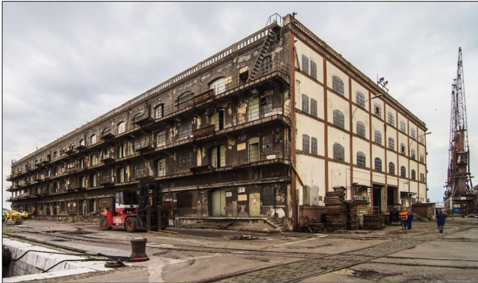
Figure 2: Front view of Warehouse no. 17 [6]
