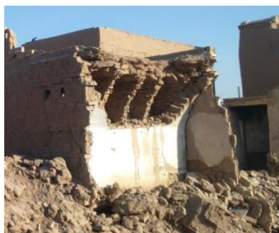
Figure 1: An example of kane poush filling the haunches of a collapsed vault, Yazd (Crété, 2015)
