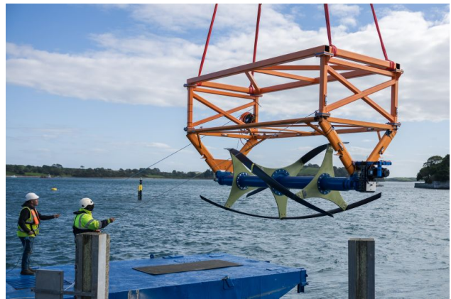
Figure 1: Deployment of the ORPC cross flow turbine in Strangford Lough in 2024, UK.
