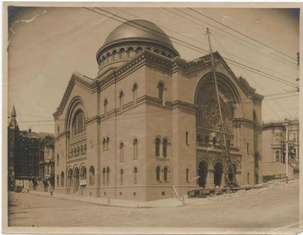
Figure 5: South cornice undergoing repair after 1906 earthquake
