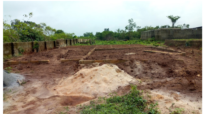
Figure 1: Soil Arrangement on Site
