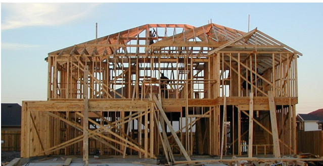
Figure 2: Use of lumber for structural framework.
