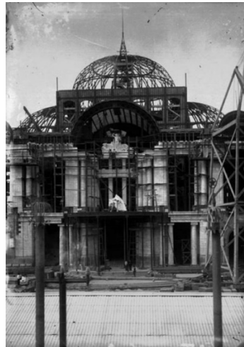
Figure 2: Construction of Palacio Bellas Artes, from Milliken Brothers Catalogue 1912.
