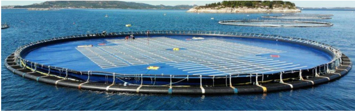
Figure 1 Floating surface tarpaulin with solar panels. (Ocean Sun 2018)
