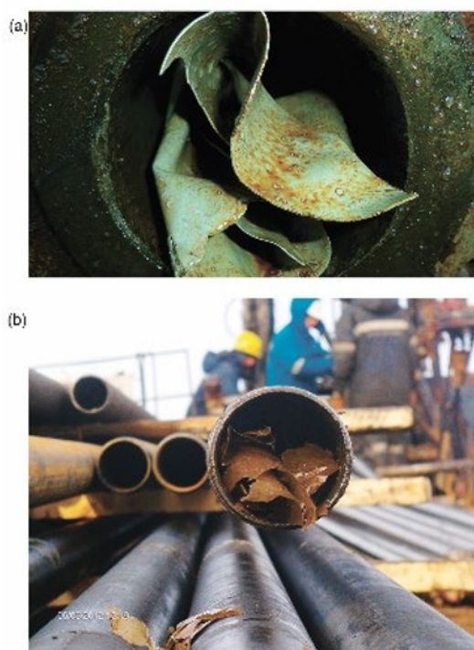
Fig. 1. Appearance of the coatings of the fielding pipe (a) and the tubing (b), destroyed by the mechanism of decompression peeling
