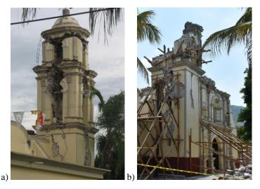
Figure 1: Damaged tower of temple of Pilcaya, Puebla: a) after earthquake; b) few days after the seismic event
