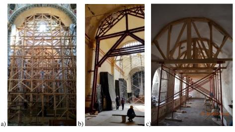
Figure 4: Examples of shoring systems: a) wood; b) steel; c) mixed
