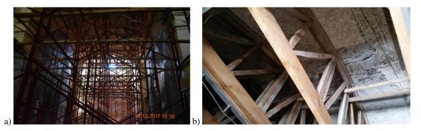
Figure 6: Example of bad criteria of emergency works: a) excessive shoring; b) shoring over a crack
