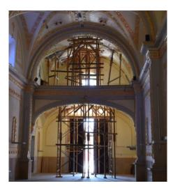
Figure 3: Example of a correct transmission of shoring system loads of higher than lower levels
