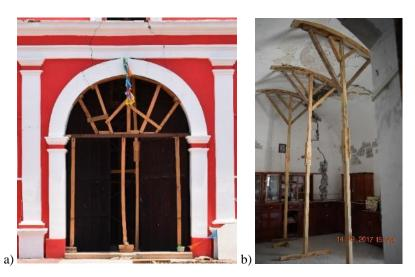
Figure 5: Example of bad quality wooden elements: a) buckled element; b) slender elements
