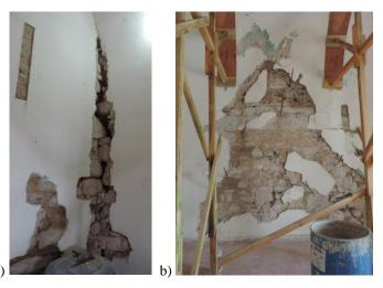
Figure 9: Damage on walls of a cloister: a) cracks; b) consolidation of the cracks
