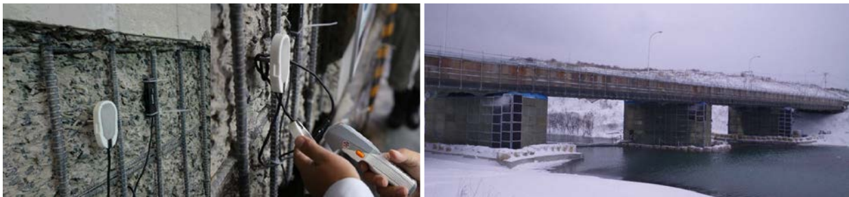
Figure 8. Application of the system to bridge pier repairs.
