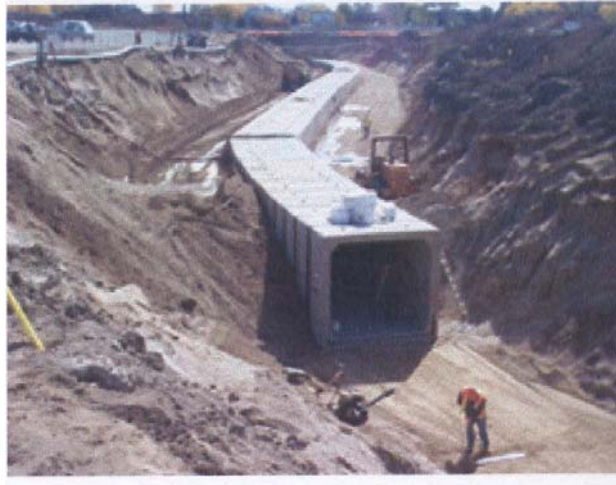
Figure 2.2.8 Large box culvert made of reinforced concrete that can be used for constructing large rectangular conduits for PCP using the open-cut construction method. (Photo reprinted from the web page of the Hanson Pipe & Products, Inc. [10])
