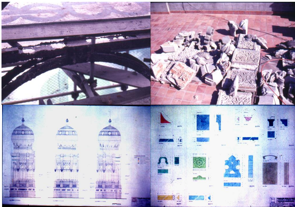
Figure 4. Interventions on the Manguinhos Historical Architectural Ensemble. From left to right: metallic structure, ornaments made of cement and sand, drawings of the façades, and ornaments of the towers of the Moorish Pavilion (1990s). DPH-COC-Fiocruz archives. Photograph by Benedito Tadeu de Oliveira
