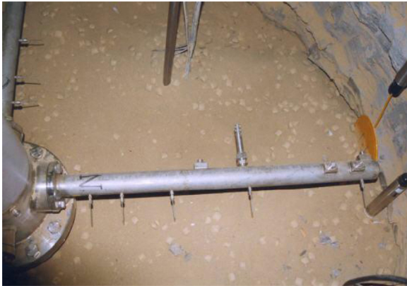
Fig. 10. Shaft backfill with a mixture of bentonite pellets and bentonite powder.
