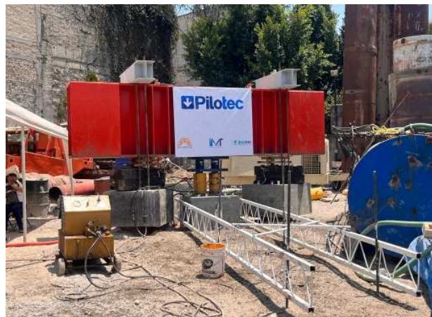
Figure 10: Arrangement for compression load test
