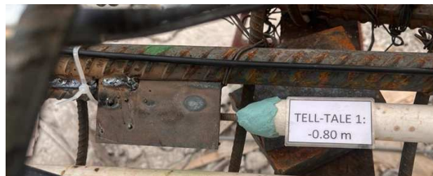
Figure 12: Placement of tell-tales in micropiles
