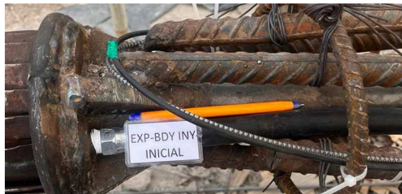
Figure 11: Embedded DFOS placement.
