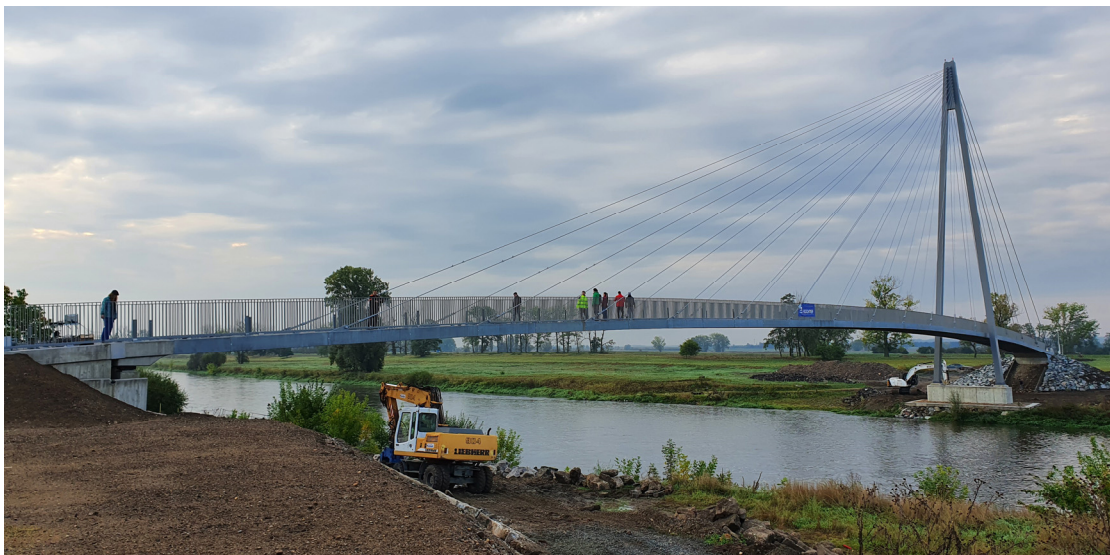
Figure 5: Suspended footbridge at Lužec-Bukol
