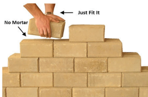
Figure 8: IMMWs mechanism [94]. Adapted with permission from Ref. [94]. Copyright ©2023, Sciepub
