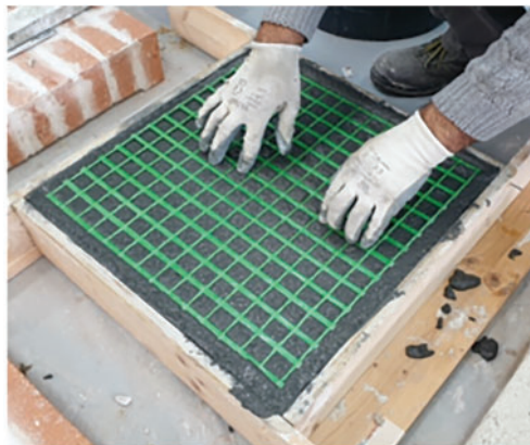
Figure 13: Textile reinforced mortar (TRM) and fabric reinforced cementitious matrix (FRCM) retrofitting techniques [134]. Adapted with permission from Ref. [134]. Copyright ©2021, Springer
