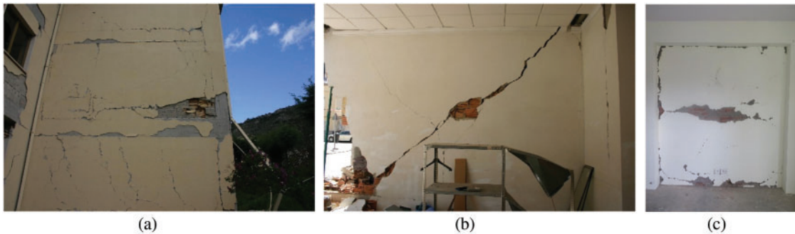
Figure 3: Common types of damage in IP IMWs: (a) separation from the surrounding RC frame due to earthquake in Italy, (b) diagonal cracks observed in Lorca, Spain, and (c) damage recorded during the Nepal earthquake [56]. Adapted with permission from Ref. [56]. Copyright ©2016, Elsevier B.V.
