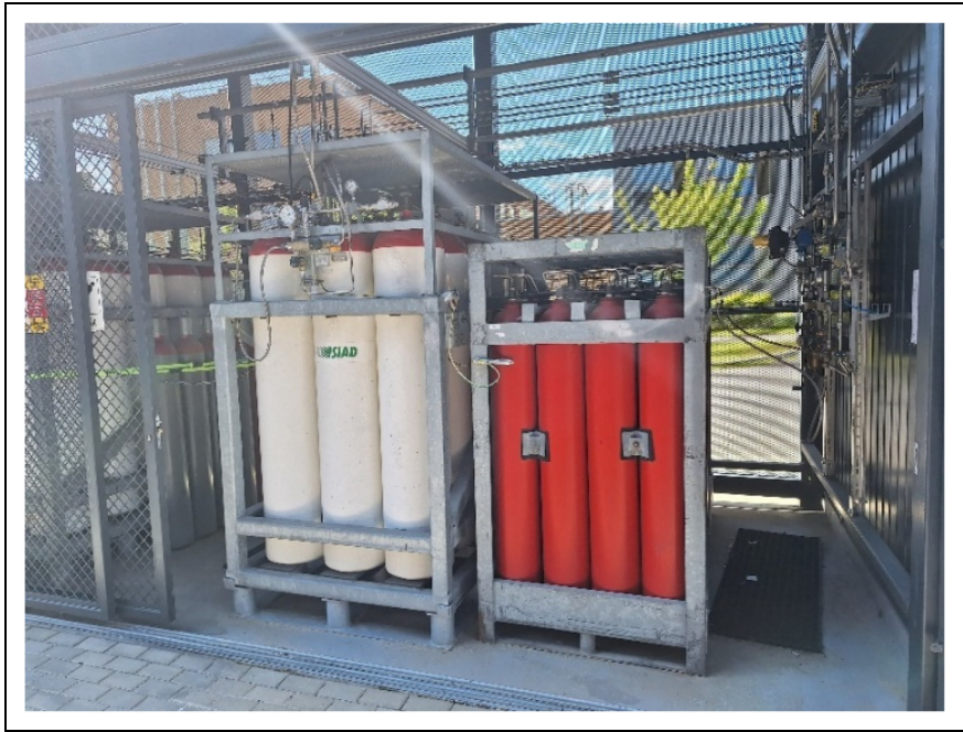
Figure 14. Hydrogen storage tanks installed in the gasification facility.
