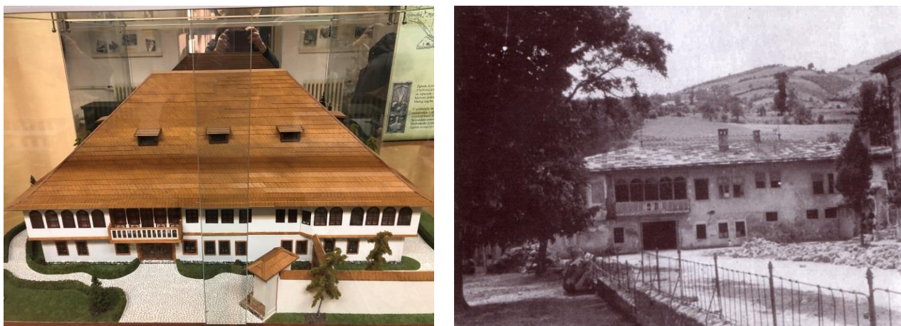
Figure 1: Left: Reconstruction model of the konak building in Travnik under Ottoman rule, with the traditional Bosnian steep roof silhouette, wooden roof-cover and hatches for the smoke ( photo Jaeger-Klein, May 2019 ); Right: The building in 1950 with the gently-sloped roof, the fire-proof brick covering and chimneys according to the regulations of Austro-Hungarian administration ( photo from Sujoldžić, Stari Vodovodi, 2012, p.94 )
