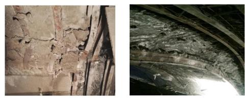
Fig. 1 Distortion and deformation of on-site steel frame support
