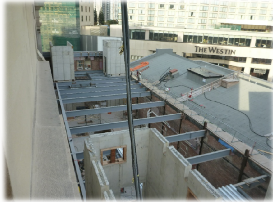
Figure 6: looking down at Ticketing Block from NW corner
