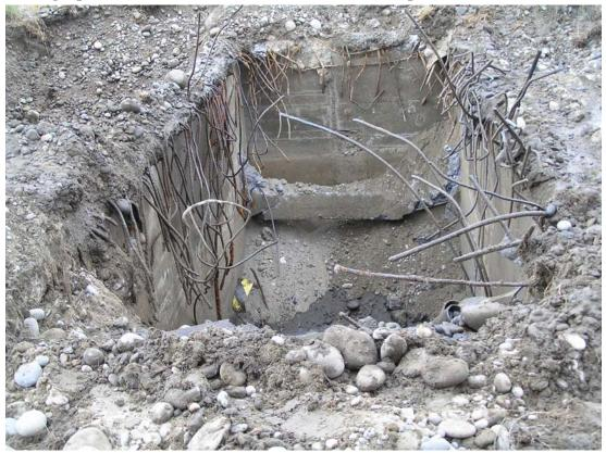
Photograph A-2. Excavation to Bottom of 1607-B1 Septic Tank (taken 5/21/07).
