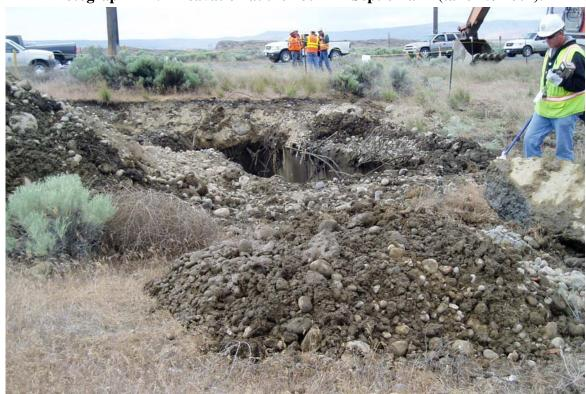
Photograph A-1. Excavation at the 1607-B1 Septic Tank (taken 5/21/07).
