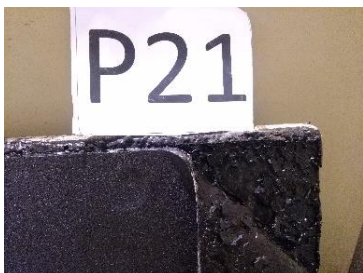
Figure 8. Debonding of the bituminous sheet of the substrate with increase the temperature.
