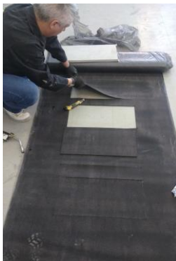
Figure 1. Preparation of Bituminous sheet.
