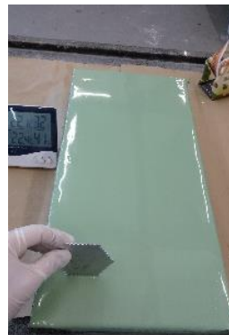
Figure 3. Application of Polyurethane membrane and inspection the thickness.
