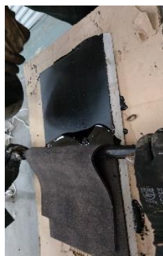
Figure 2. Application of the Bituminous sheet adhered with heated cement asphalt.
