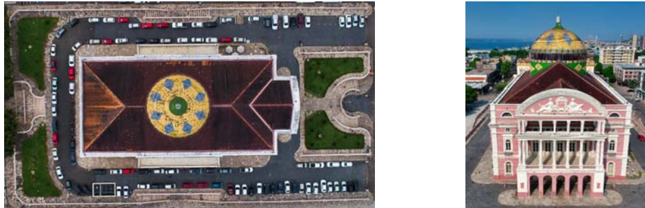
Figure 3: Amazonas Theater: a) Upper View; b) Frontal facade. Photo by Ivo Brasil Filho on June 4, 2019 [17].
