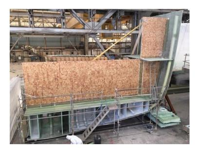
Demonstrator currently under construction at iXblue showing **laminate** and **sandwich** construction
