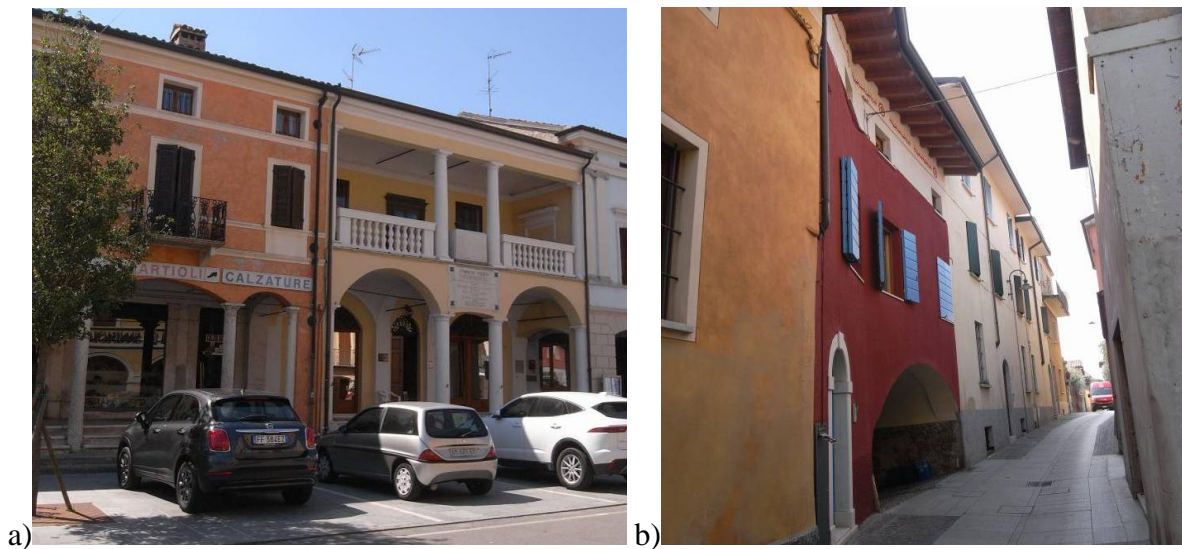
Figure 3: Fragilities in the structural units: a) porch and b) covered walkways.
