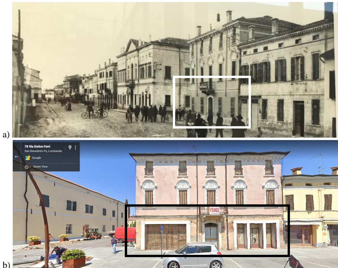
Figure 2: Transformations: a) XX century image of a traditional Italian historical center with the detail of a three storey building, b) widening of the original openings, compromising resistance to horizontal actions.
