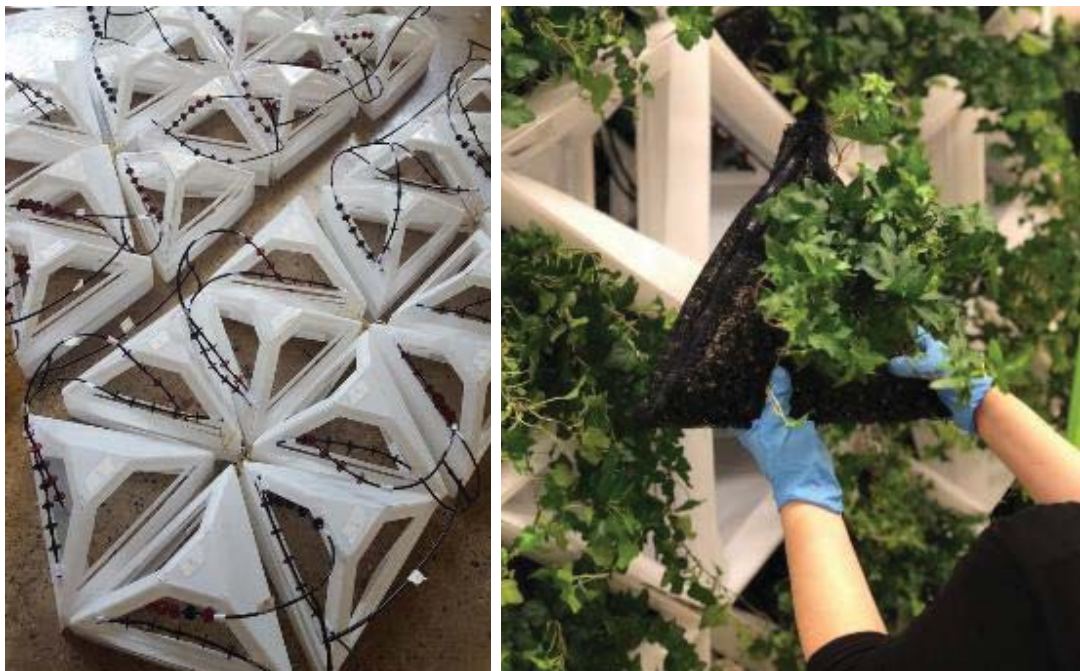
Figure 3. a. Folded cassettes and dripper attachments; b. 3d mesh holding growing media and plants.
