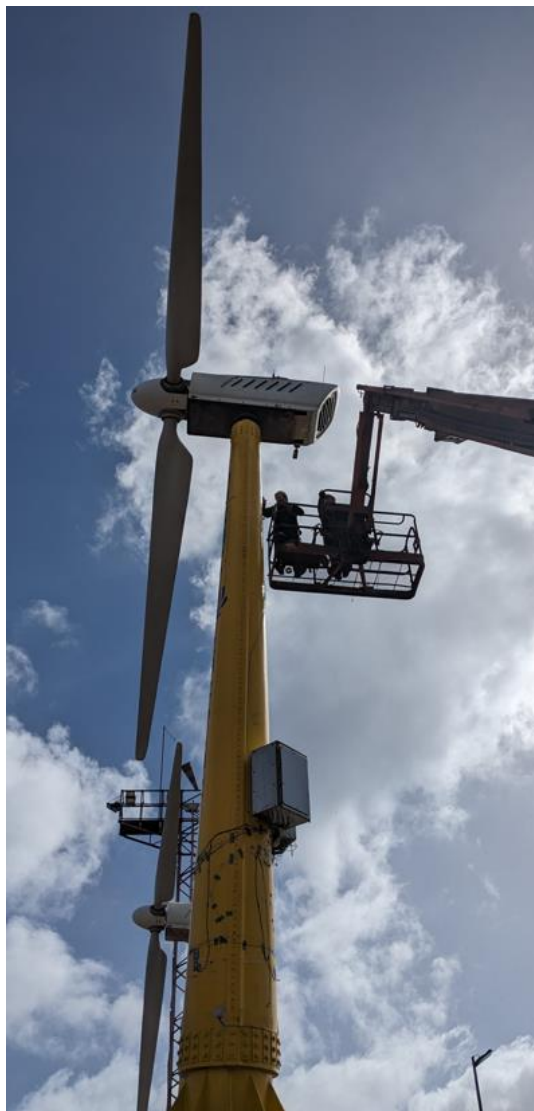
Figure 18 TSI installing the FRP monitoring system.
