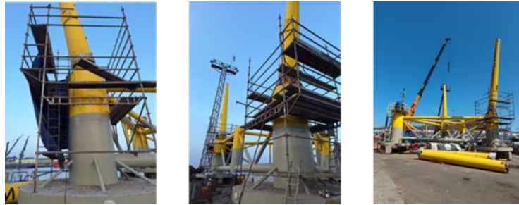
Figure 5 Lifting and assembly of the FRP towers.
