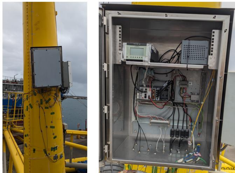
Figure 23 Monitoring cabinet installed at the tower.
