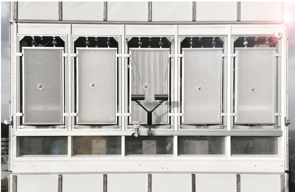
Figure 1 HydroSKIN façade prototypes at D1244 experimental high-rise building in Stuttgart © Christina Eisenbarth
