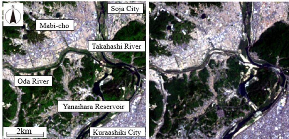
Fig. 1 Satellite image data (left : before the disaster, right : after the disaster)
