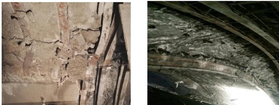
**Fig. 1** Distortion and deformation of on-site steel frame support
