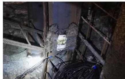
**Figure 5** Schematic diagram of welding and protection of strain gauge components
