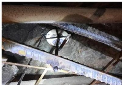
**Figure 4** Installation of the initial pressure cell
