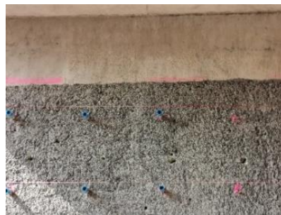
Figure 3. Visual inspection of the front wall of the bridge.
