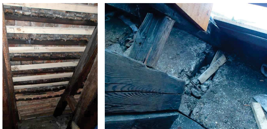
Figure 4: False rafters and reinforced timber roof truss components
