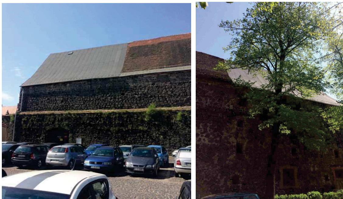
Figure 1: Temporary security after phase 1 and 2
