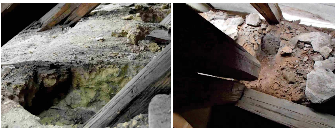
Figure 8: Pugging on the top part of the walls
