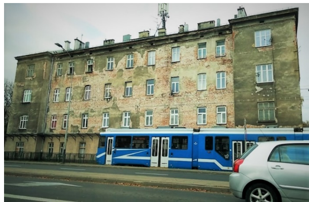
Figure 8. Tram line and busy two-lane road in the Borek Fałęcki district in Krakow, 25/10/2016.
