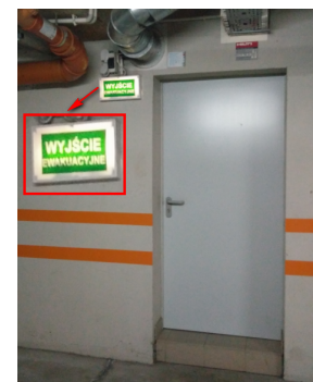
Figure 6. Emergency exit from the underground garage in a residential building 11/10/2016.
