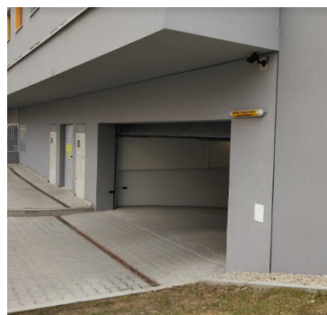
Figure 5. Entrance to the underground garage with a display informing about the concentration of carbon monoxide 12/06/2016.
