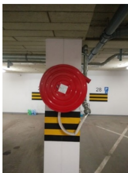
Figure 4. Fire extinguisher placed in the underground garage of a multi-family building 02/02/2016.
