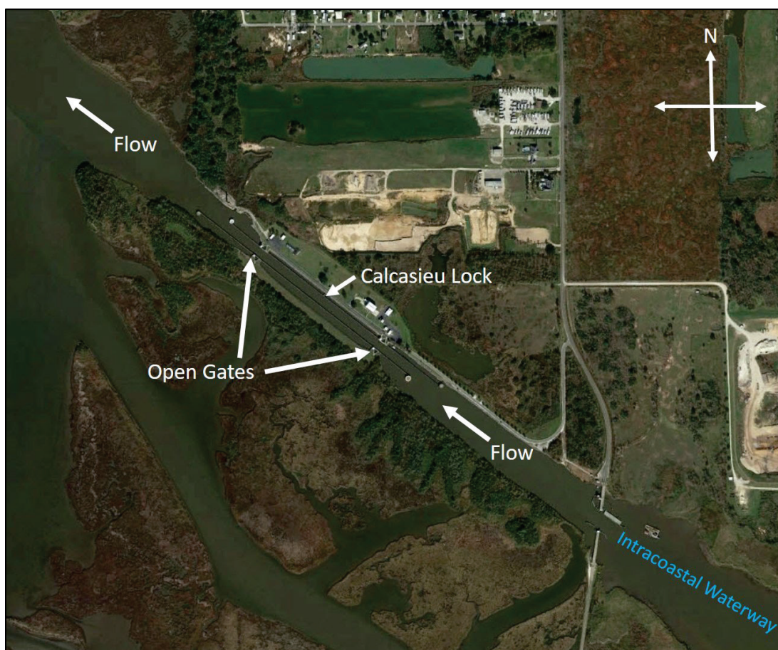
Figure 3. Calcasieu Lock during draining mode.
