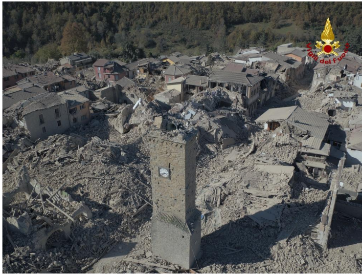
Figure 2: Amatrice historical centre, after the 24 August event in a snapshot from a movie released by the Firefighters Corps ( www.vigilfuoco.tv )
