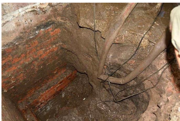
Figure 9: Exposure of the foundation walls
