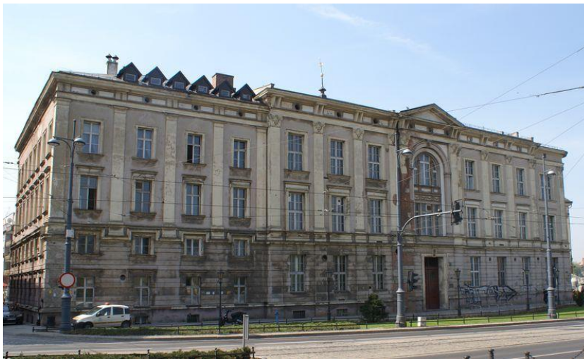
Figure 8: Current view (from north) of the front façade of the building
