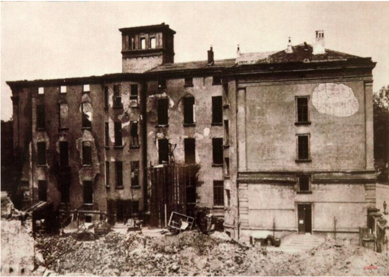
Figure 5: View of the destroyed building in 1945 (southern side) [4]
