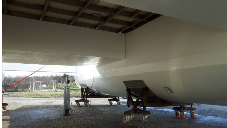
Figure 1: The bottom of the catamaran during construction
