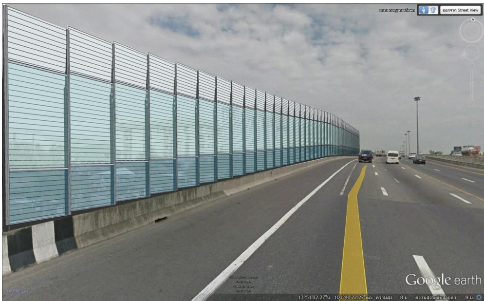
Figure 4. Noise Barrier on the Pilot Area
