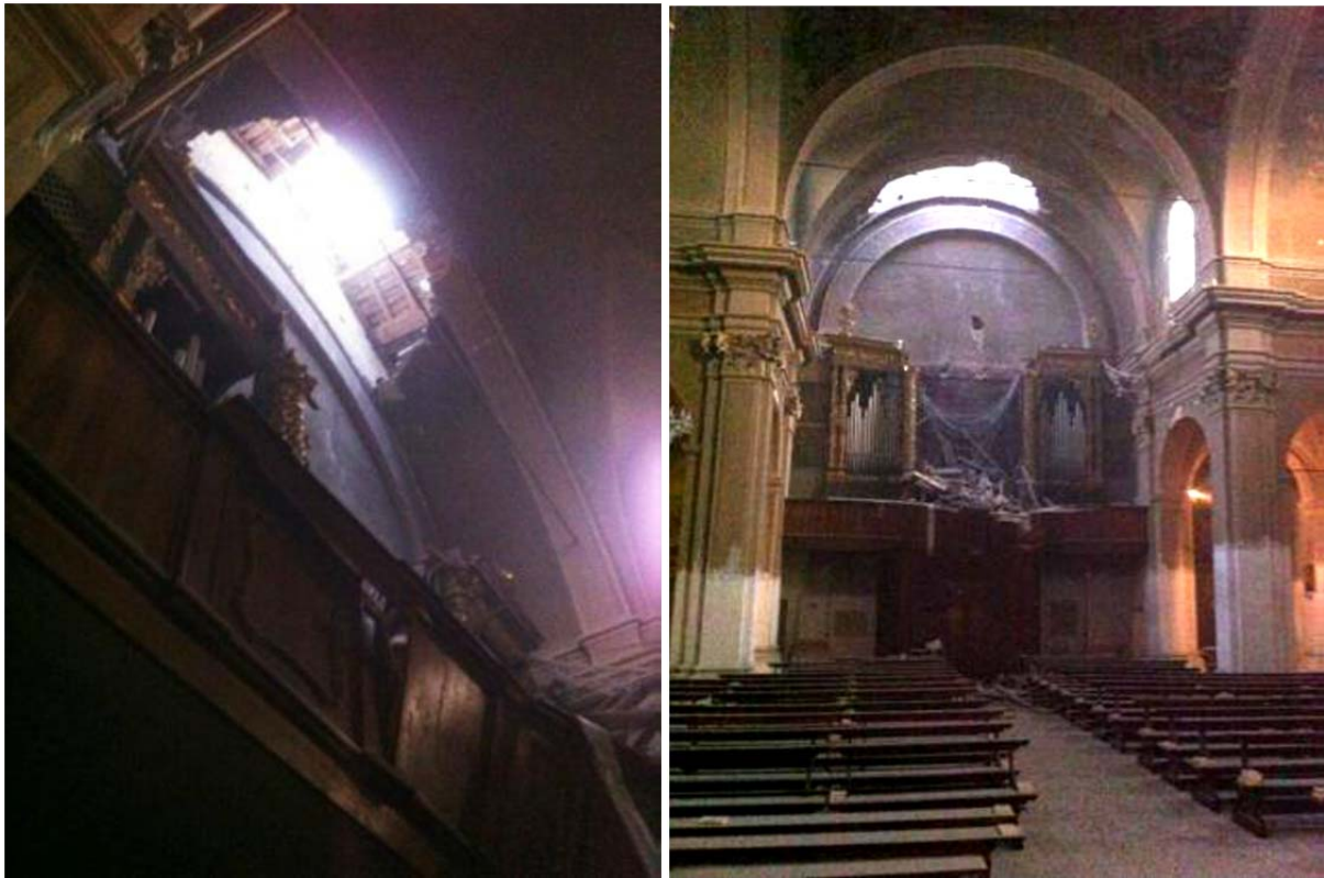
Figure 5: Collapse of the vault behind the façade
