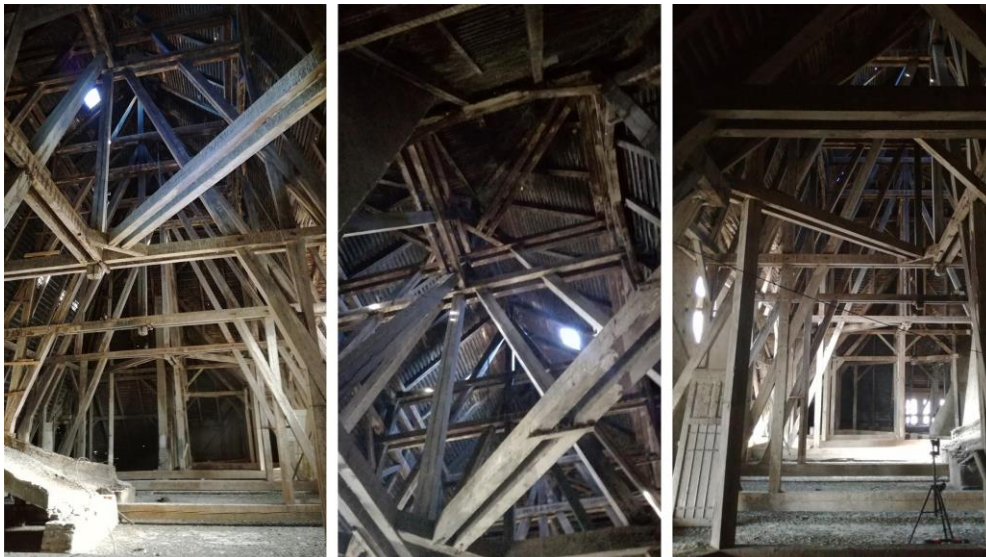
Figure 3: Roof structure above the gables
