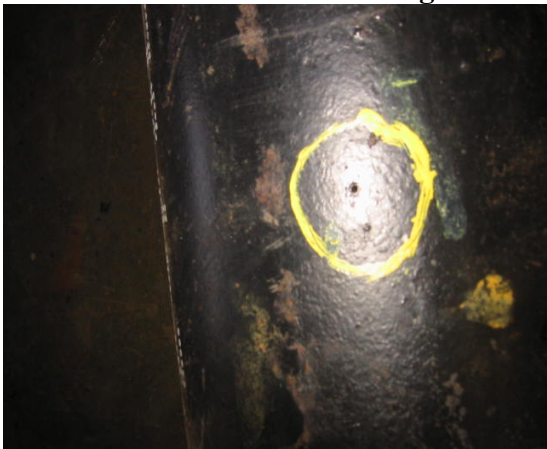
Photo 27: External View before Flex-Plug
