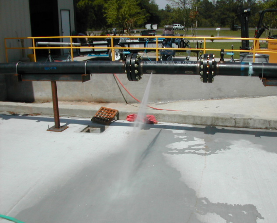
Photo 6: External Corrosion Leak Rate Testing
