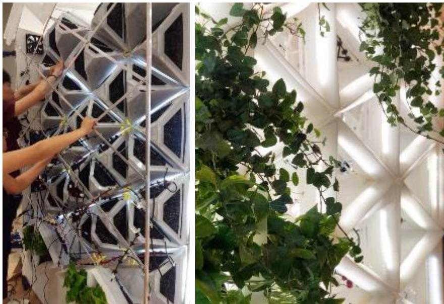
Figure 4. a. Assembly of the prototype; b. Plant assembly of the prototype.
