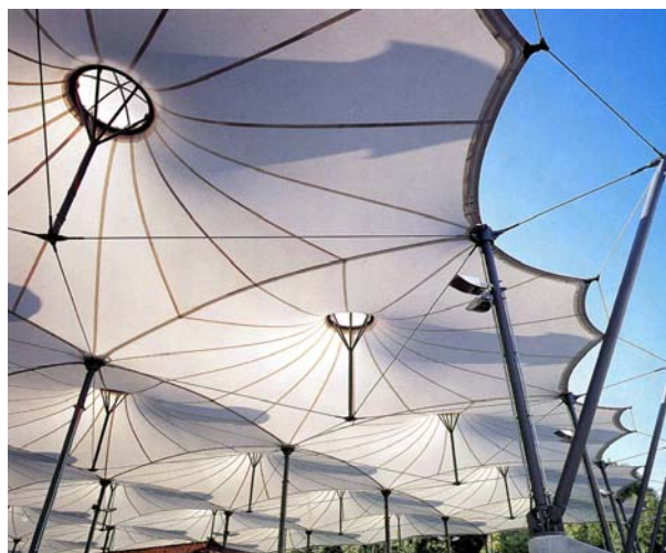
Figure 35: Waste Management Office, Munich [7]
