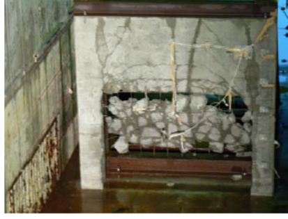
Fig. 20: Concrete wall under tsunami force. Cracked geometry of the wall after the experiment conducted in Arikawa et al. [66].
