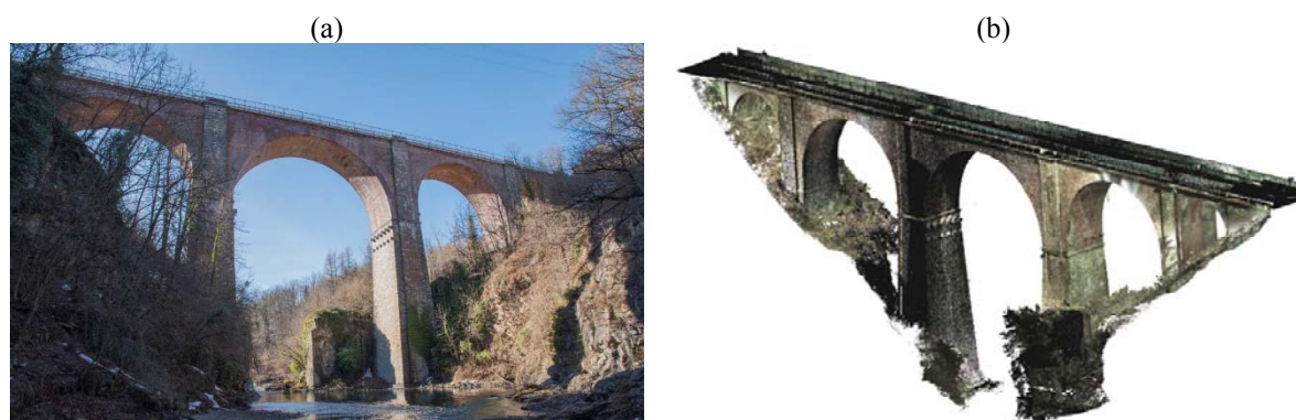
Figure 1: The Olla bridge: (a) View from the Stura river; (b) 3D model from the geomatic survey [4].
