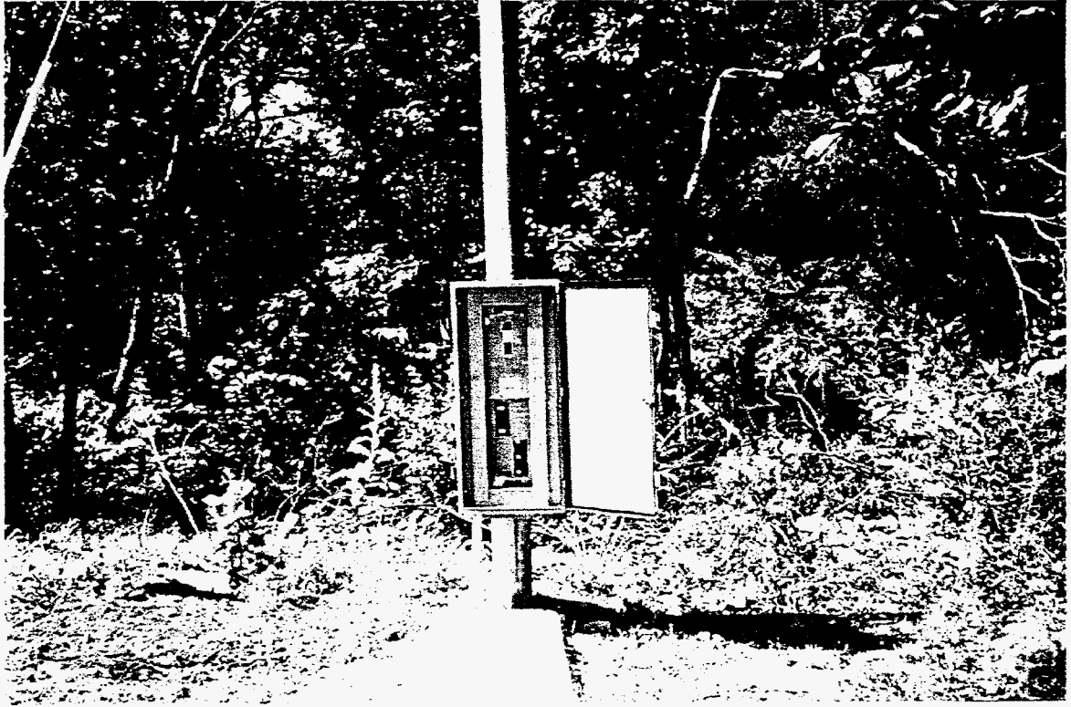
Figure 13. Main power system
