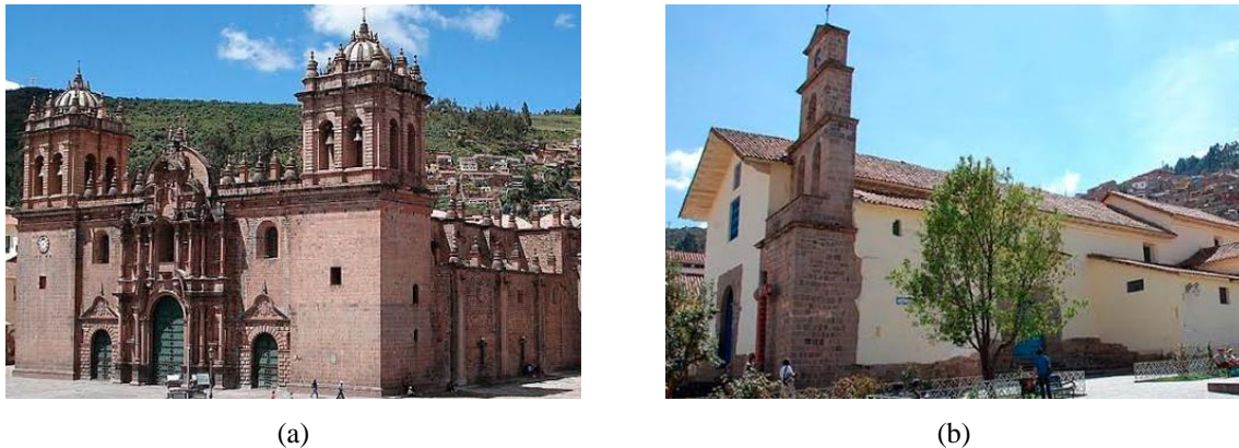
Figure 1: Materials used in Cusco churches a) Stone with lime mortar in the Basilica de la Catedral and, b) Adobe with mud mortar in the Templo de San Blas .
